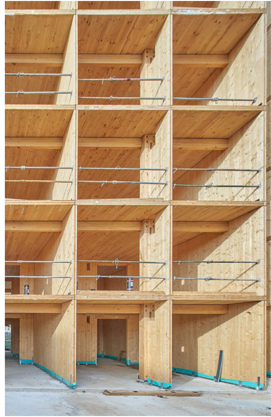
Hybrid Timber Structure (Gallery of Hybrid Timber Structure in 6-Story Building - 1, n.d.)
