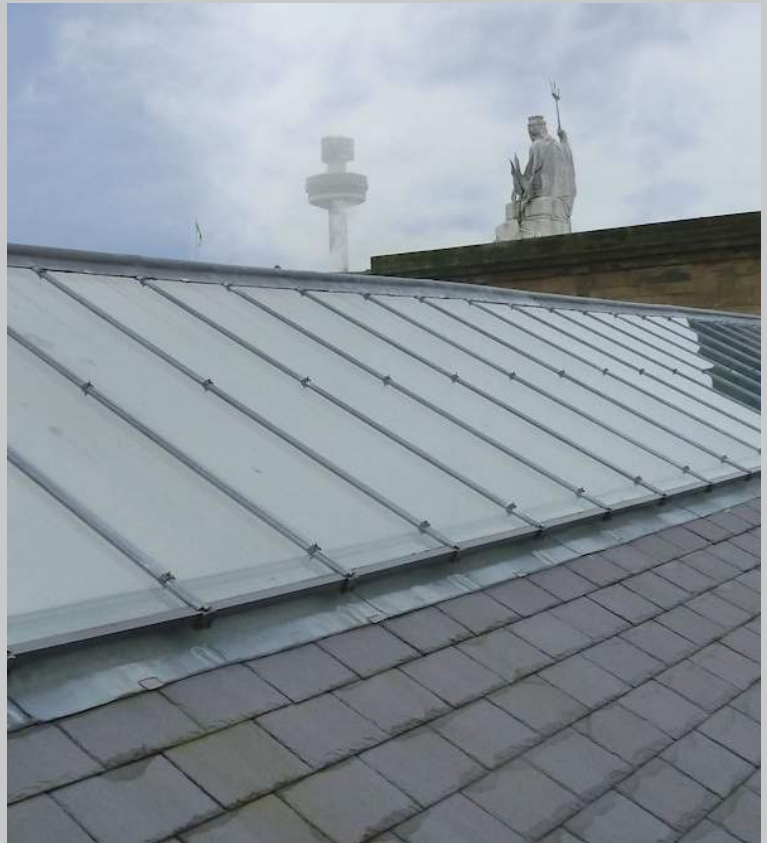
Figure 2.10-skylight with patent glazing
