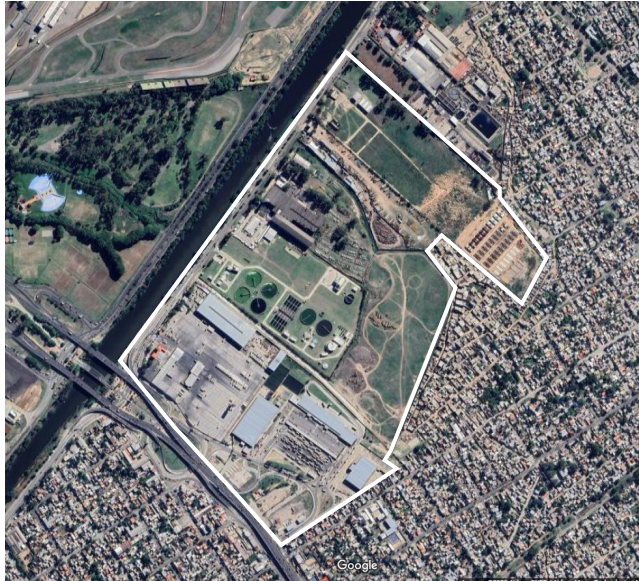
A new wastewater treatment plant in Lanus
