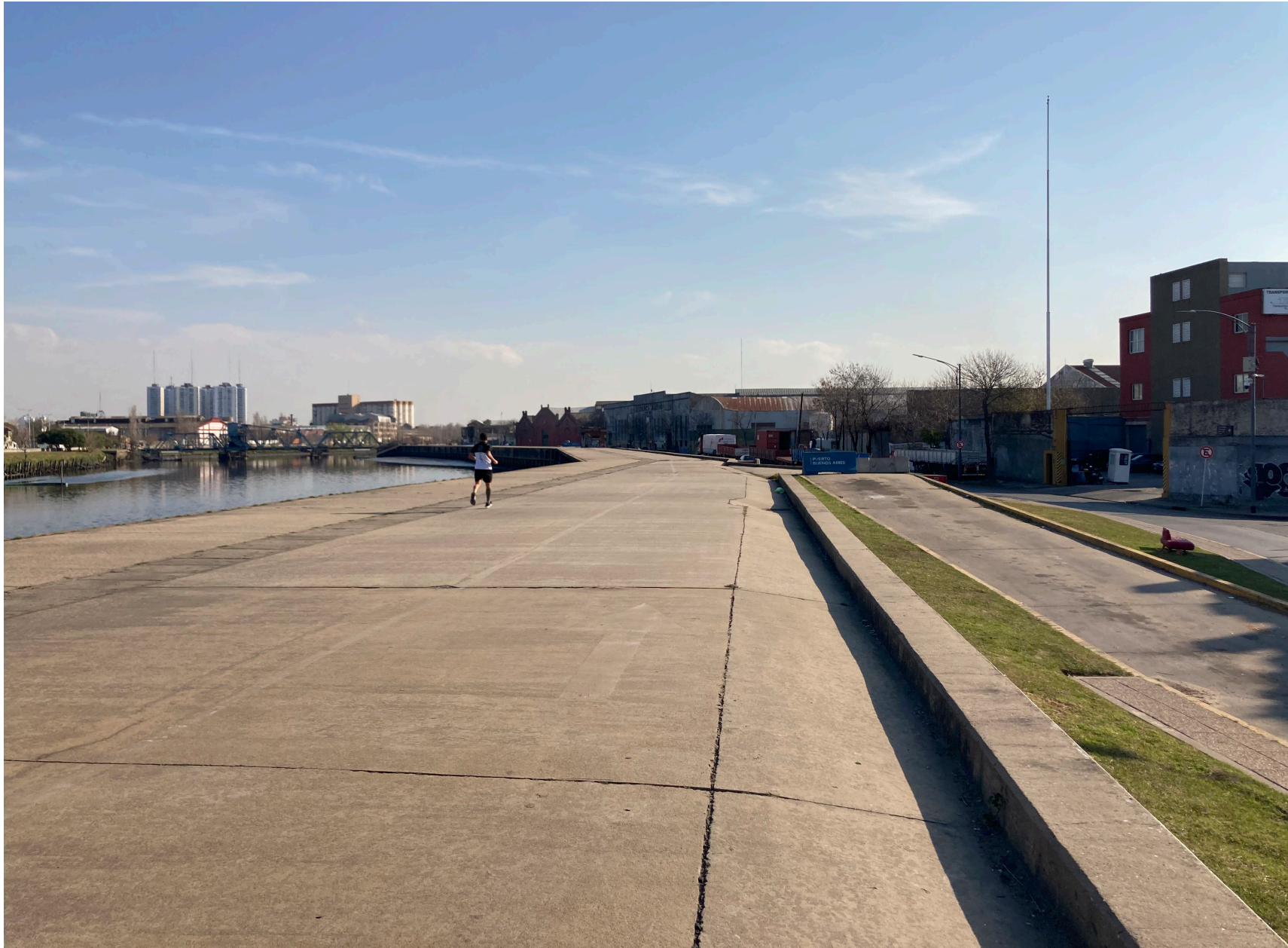
concrete along the river's edge
