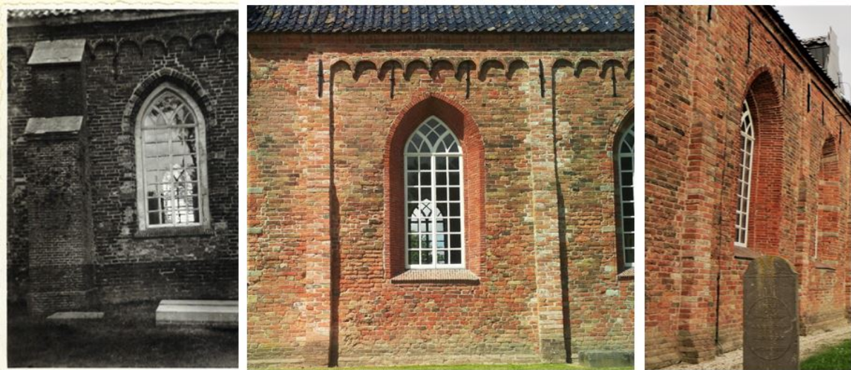
Figure 5.9: Photos the piers before (left) and after the modifications (middle and right)
