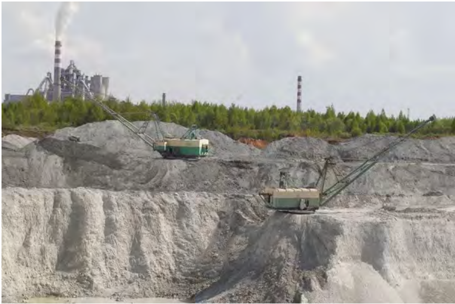
Cement Factory depositphotos.com
