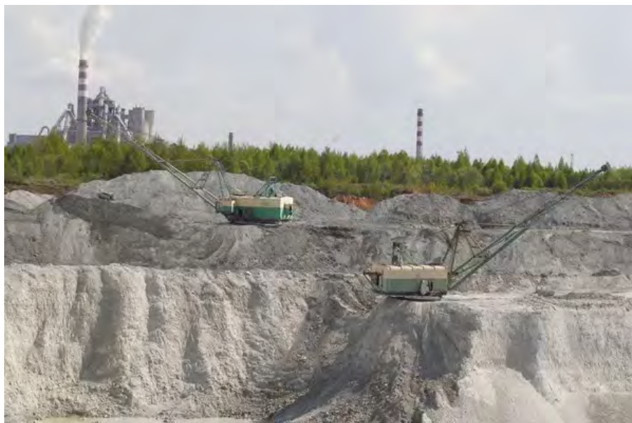
Cement Factory depositphotos.com
