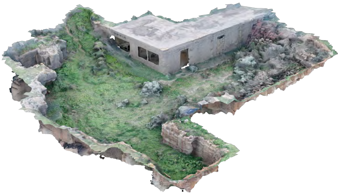
Construction Site area = 700m2/100m2 residents = abandoned
