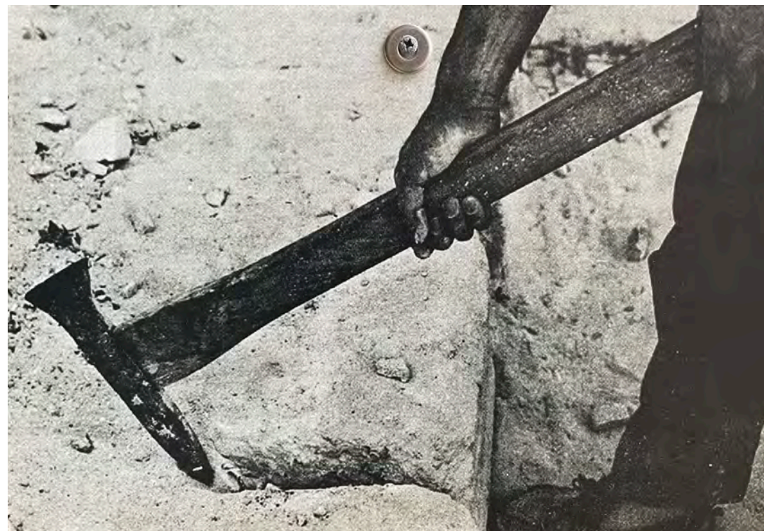
Calcarenite Quarry 19th century Manual Extraction Archived Photo - Giardino dell Impossibile
