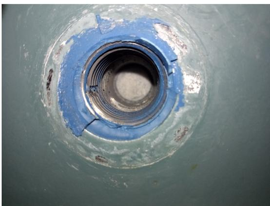
(a) Resin injected hole in the steel beam flange
