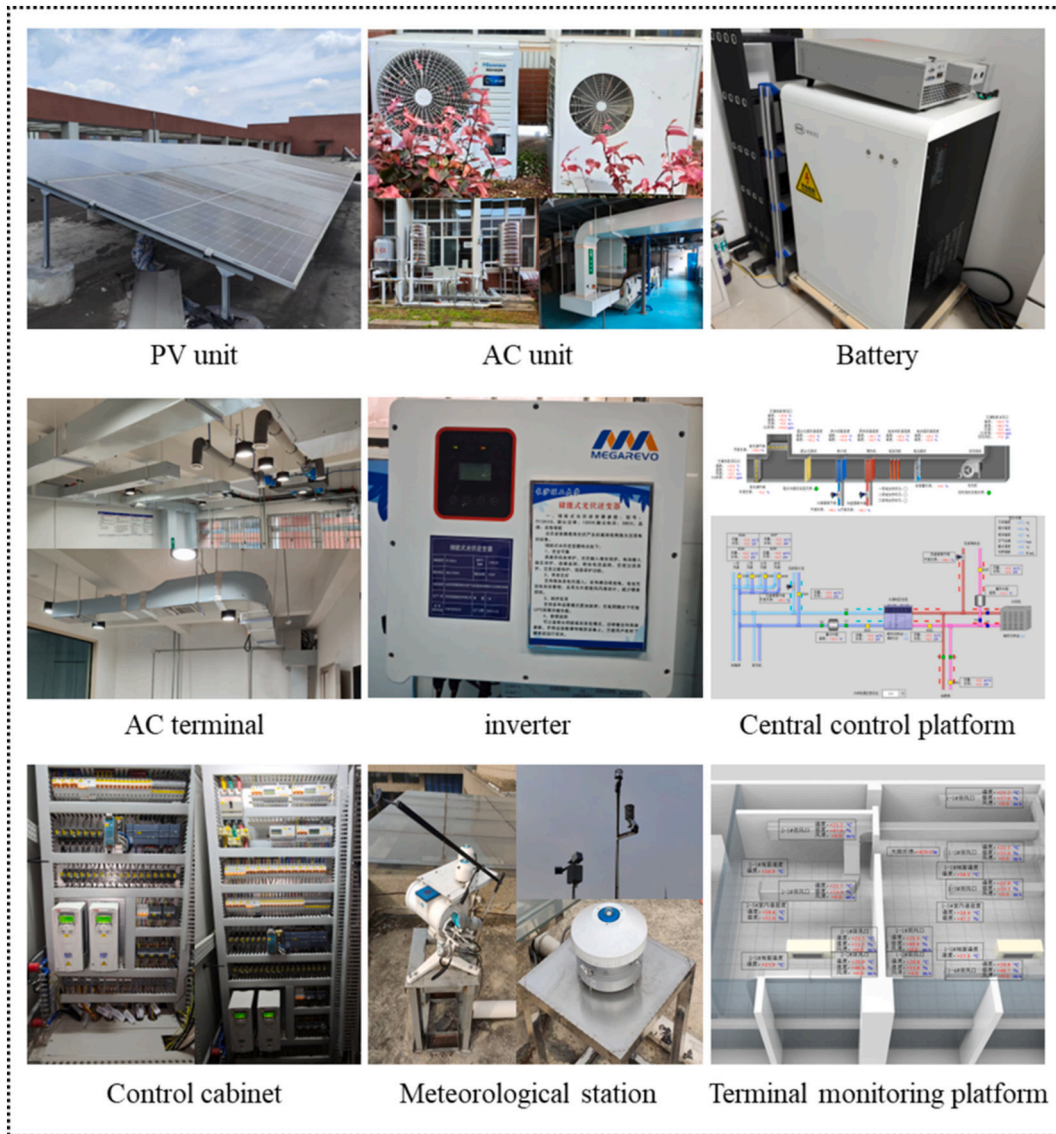
Fig. 3. PVAC experimental platform with PTPS operation model.
