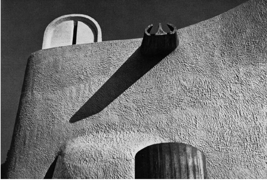
Fig. 9 Le Corbusier: Gargoyle on the Façade of Notre-Dame du Haut, Chapel in Ronchamp, France, 1955
