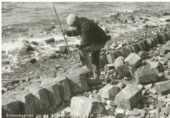
Figure 1-1 Traditional Basalt column revetment construction at Afsluitdijk, 1931
