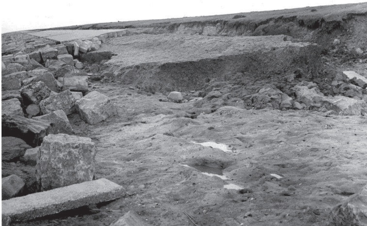
Figure 2-16 Photographs of damage to stretches of the Afsluitdijk near Wieringen, February 1953
