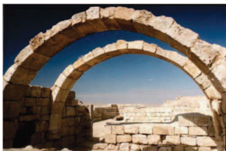
Figure 3–14 Examples of compressed not-bonded joints
