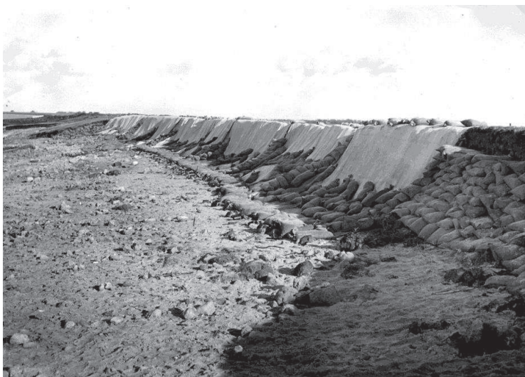
Figure 2-14 Photograph of damage to the dike and the emergency repairs at the North side of Wieringen, near Hypolytushoef, February 1953
