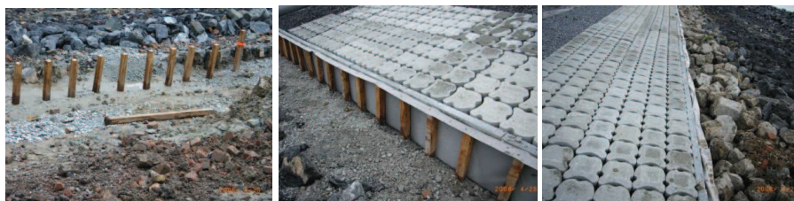
Figure 3–24 Photographs of construction of toe structure type (b) at Schouwen-Duiveland in 2008
