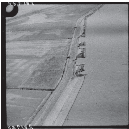
Figure 2-14 Photograph of damage to the dike and the emergency repairs at the North side of Wieringen, near Hypolytushoef, February 1953
