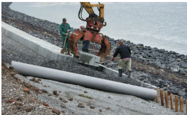
Figure 1-2 Modern column revetment construction Noord Beveland, 2008
