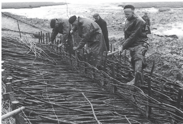
Figure 2-5 Photograph of wicker mattresses as slope protection, source: (Kool-Blokland, 2003), pp 122
