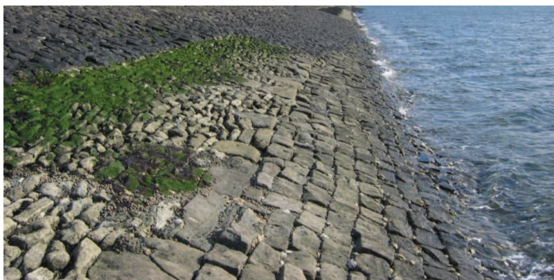
Figure 2-6 Photograph of a natural stone slope, patch work of block stone, Vilvoord stone and Basalt columns
