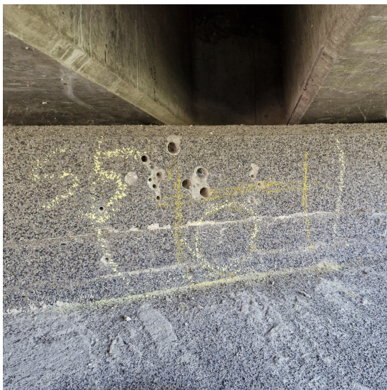
(c) Existing boreholes from previous experiments at location S5
