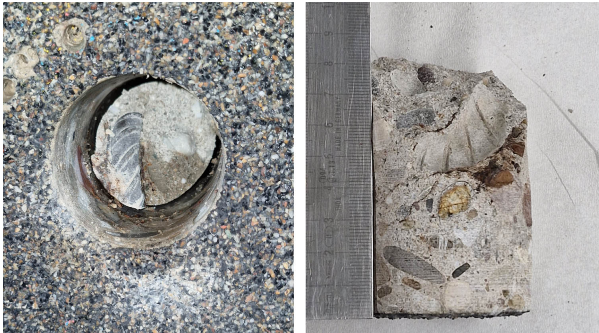
Figure 5.10: Location of S1* showing signs of corrosion products.
