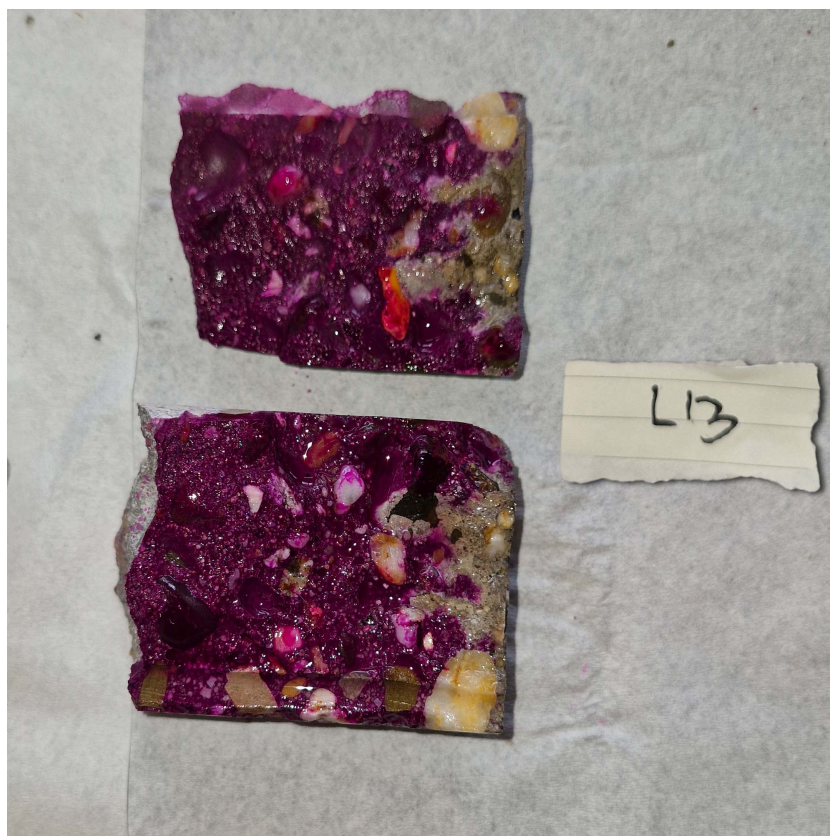
Figure F.7: Carbonation of core L13-CL1
