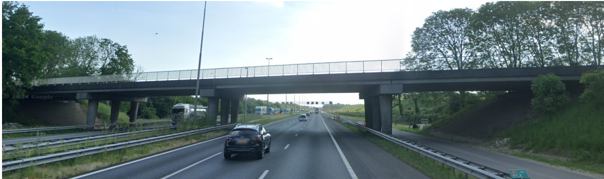
Figure 3.4: View of the Ardeweg viaduct as seen from the A1 heading to Deventer. The Aerdenbroek access road can be seen on the right.
