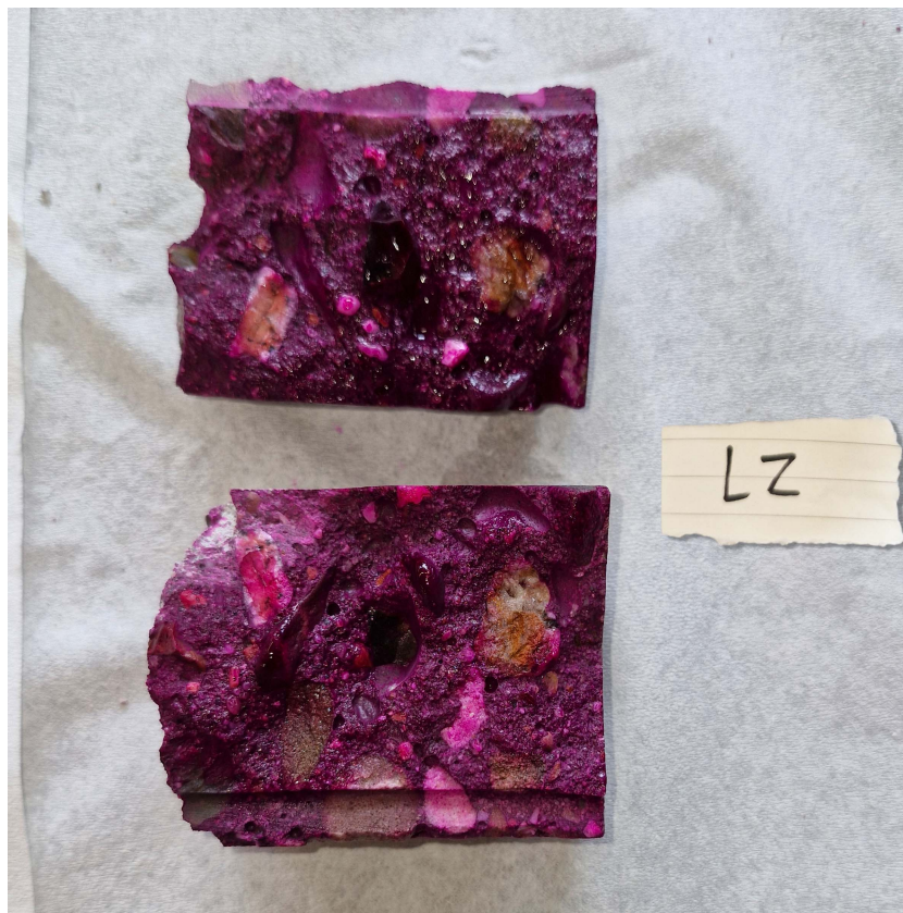
Figure F.6: Carbonation of core L2-CL1
