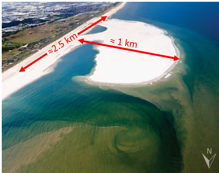
Figure 5.1: Aerial photograph of the Sand Motor after completion (September 2011). Note the clouds of fine-grained material moving to the North. Picture courtesy of Rijkswaterstaat / Joop van Houdt
