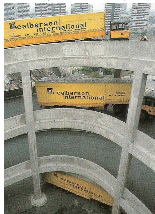
Ramps of Entrepôt Ney image retrieved from image retrieved from icade.fr on 07-05-14
