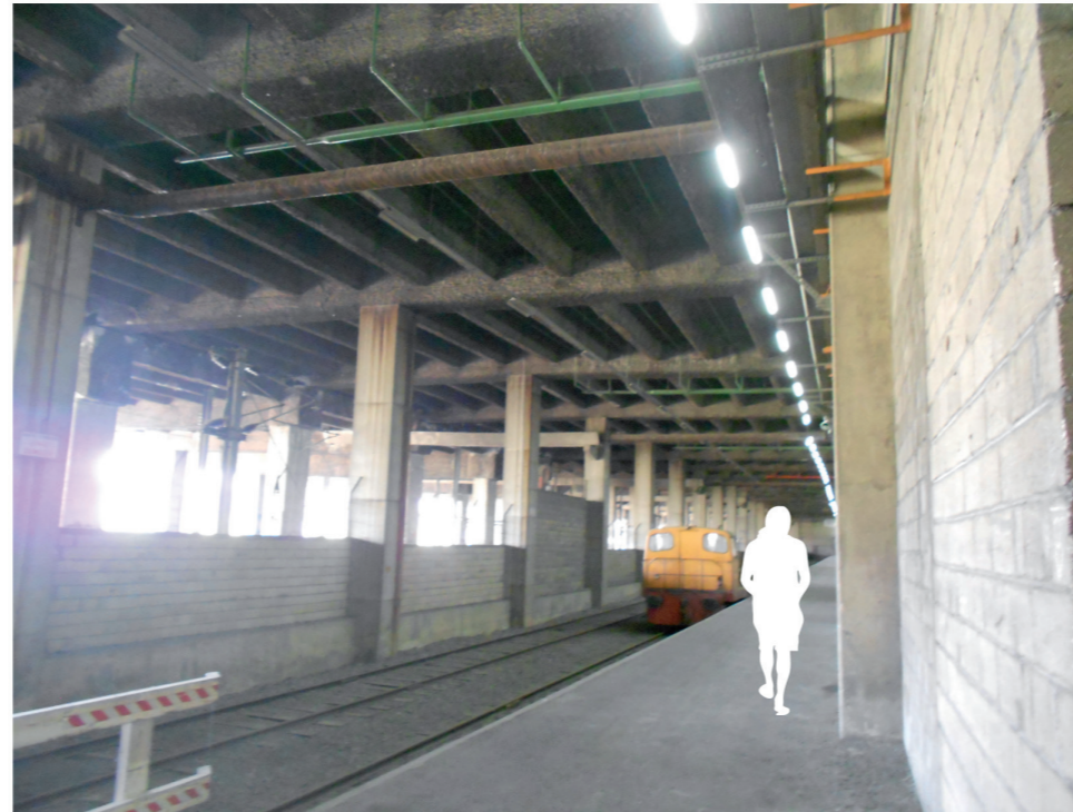
Rail platform on ground floor
