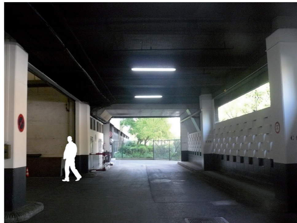
Interior route on ground floor
