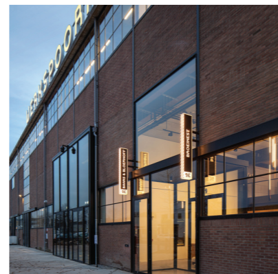
Werkspoor Factory Utrecht, Netherlands Industrial warehouse Business, Multifunctional space, Cafe, Office
