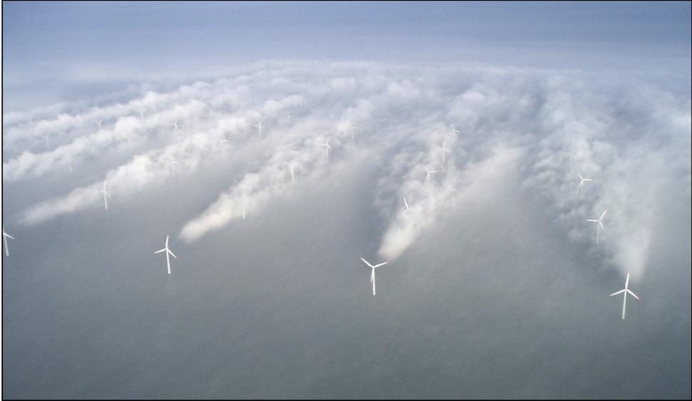
Figure 1.3: A photograph by C. Steiness of the Horns Rev wind farm off the coast of Denmark in foggy conditions (Hasager et al., 2013). These unique atmospheric conditions allow us to see wake formation and wake interaction that are otherwise invisible under normal weather conditions.
