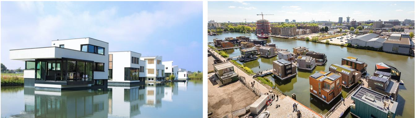
Figure 2.2: Floating structures for urban purposes. Projects Harnaschpolder, Delft (left), adapted from Blue21 (2023b) and Schoonschip, Amsterdam (right), adapted from Stedenbouw (2019)
