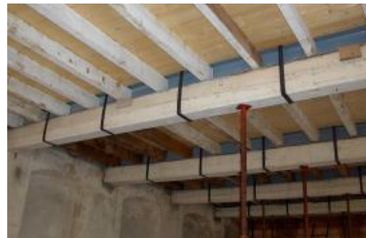
Figure 77. Reinforcement of a timber beam (Corradi et al., 2019)
