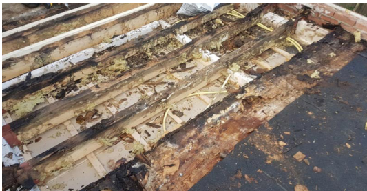
Figure 75. Wood Rot (Dak Discounter, n.d.)
