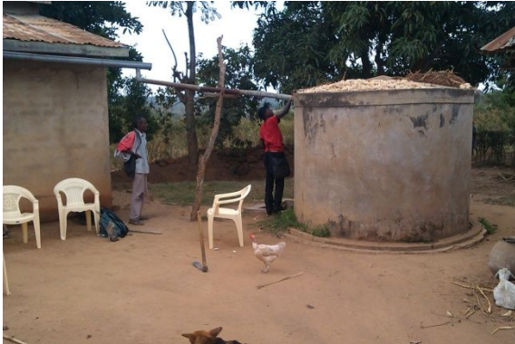
Figure A.73 Roof water harvest tank
