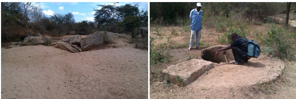
Figure A.14 Sand dam 10 (left) and well nearby (right)
