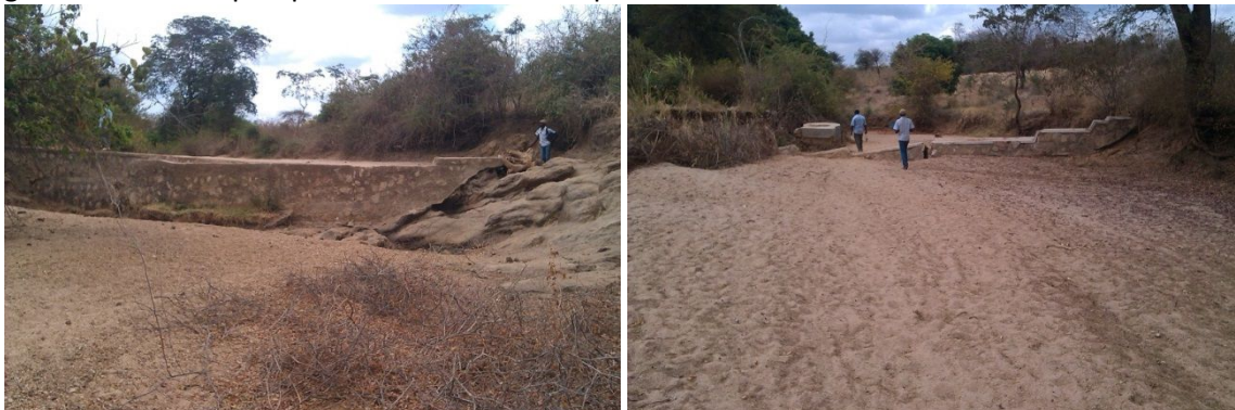
Figure A.32 Sand dam V (Left) and Sand dam VI (Right) sponsored by a donors
