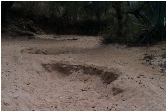
Figure A.43 Riverbed upstream of sand dam 12
