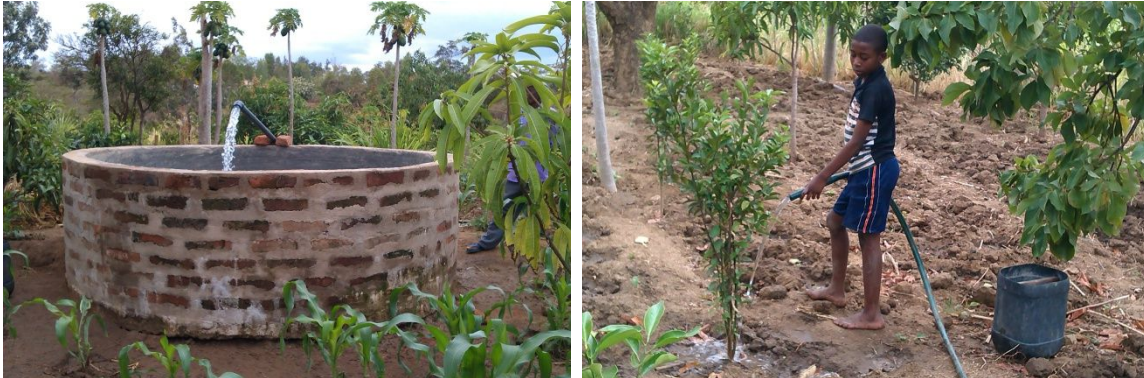
Figure A.81 Water tank (left) to irrigate vegetables by gravity with a garden hose (right)
