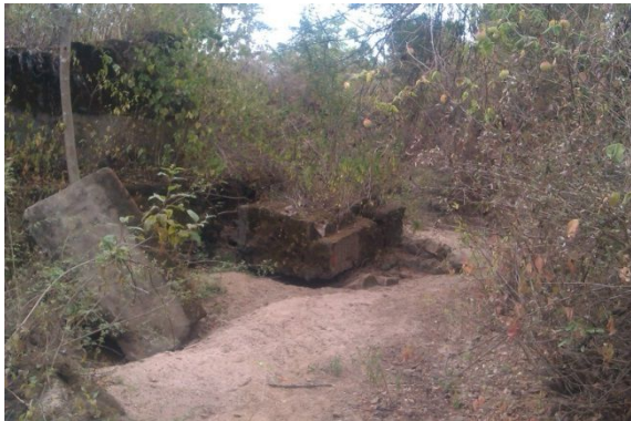
Figure A.7 Ancient sand dam
