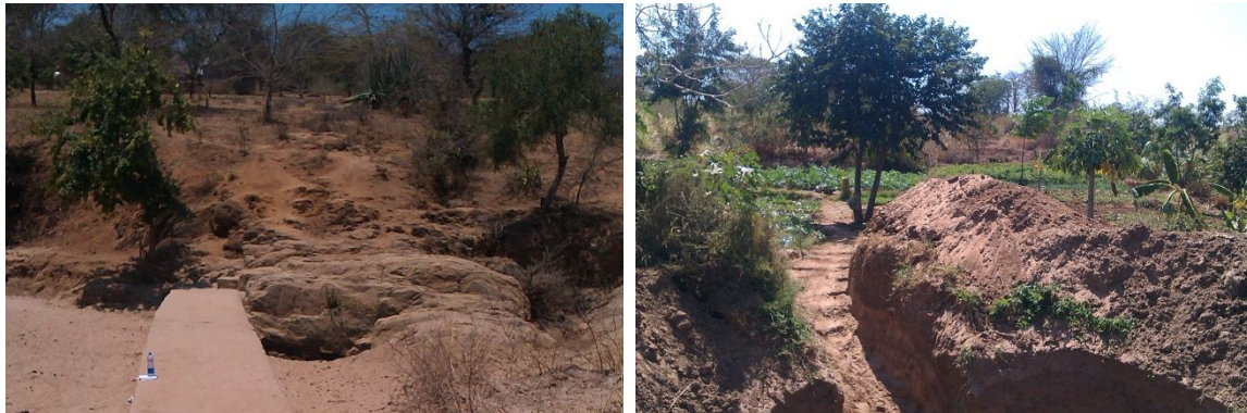
Figure A.63 Left: dry vegetation next to sand dam 18; Right: irrigated plots
