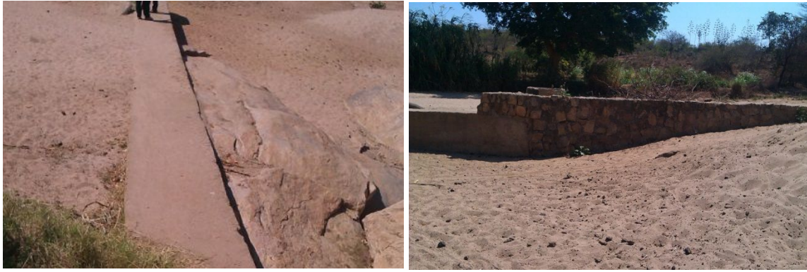
Figure A.25 Sand dam 19 (left) with extended wing wall (right)
