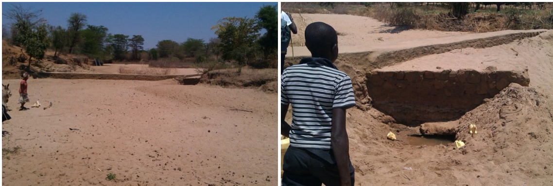
Figure A.23 Sand dam 18 (left) with repaired wing wall (right)
