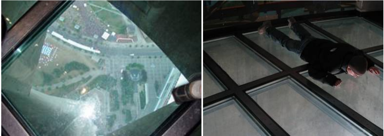
Figure 78, Steel framed glass floor of CN Tower in Toronto at 342m above ground level.
