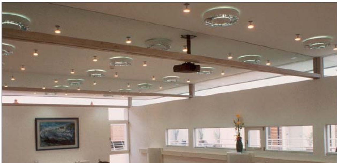
Figure 43, Timber-Glass composite beam in conference room of Hotel Palafitte in Neuchatel. [24]
