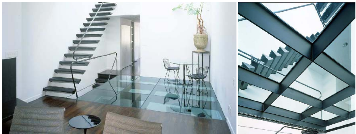
Figure 77, Steel framed glass floor seen from above (left) and underneath (right). [www.productanddesign.com]
