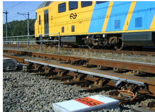
Figuur 2.4 Gas lintelement (Wikipedia, 2010a)
