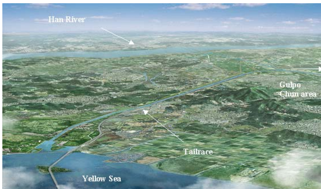
Figure A.1-1 Birthview on the Tailrace drainage channel [208]
