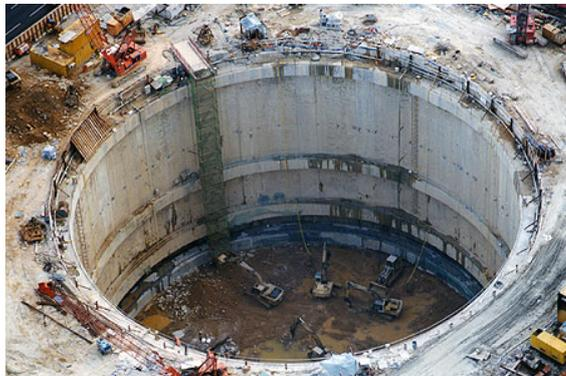
According to Kurian, 2013, diaphragm walls as can be understood from their names, are relatively thin soil retention structures embedded in soil. They are constructed in panels. At each panel, excavation of the trench, supporting of the trench with slurry, placement of the reinforcement cage, and filling of the trench with structural concrete, are executed.
