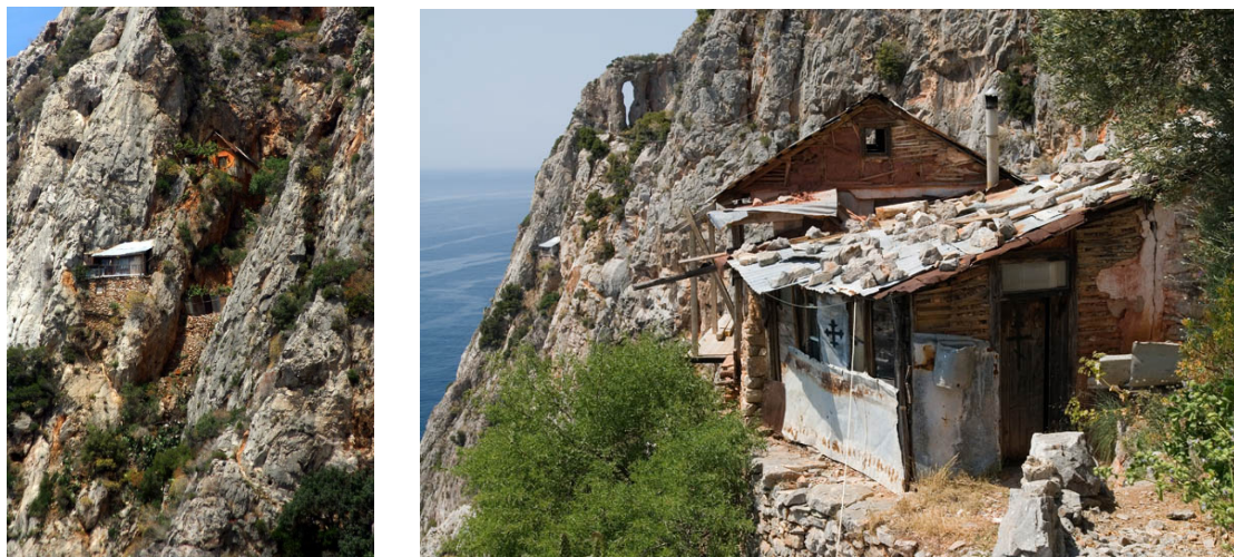
Figure 26: Hermits' Huts in Karoulia area, the southernmost area of the peninsula, Vlasis Vlasidis 2020 21 , the huts showcase construction techniques of the early 20 th century (wooden walls) and repairs with modern day metallic materials, showcasing the long history of these ephemeral dwellings.
