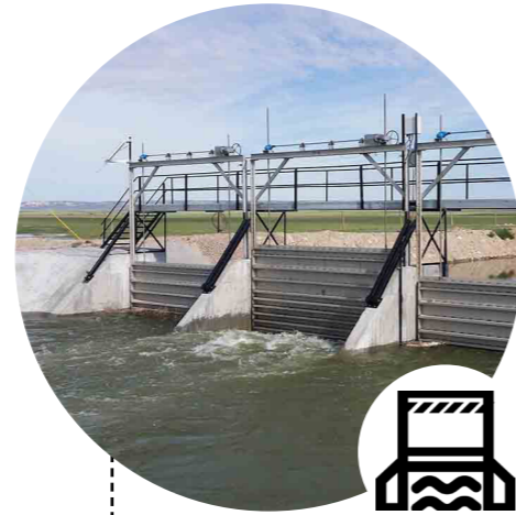
Reservoir lock + threshold
