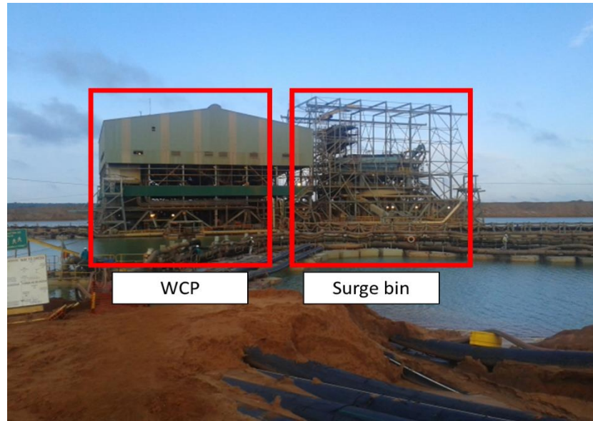
Figure A-1: Wet concentrator plant (left) and surge bin (right) in Mozambique
