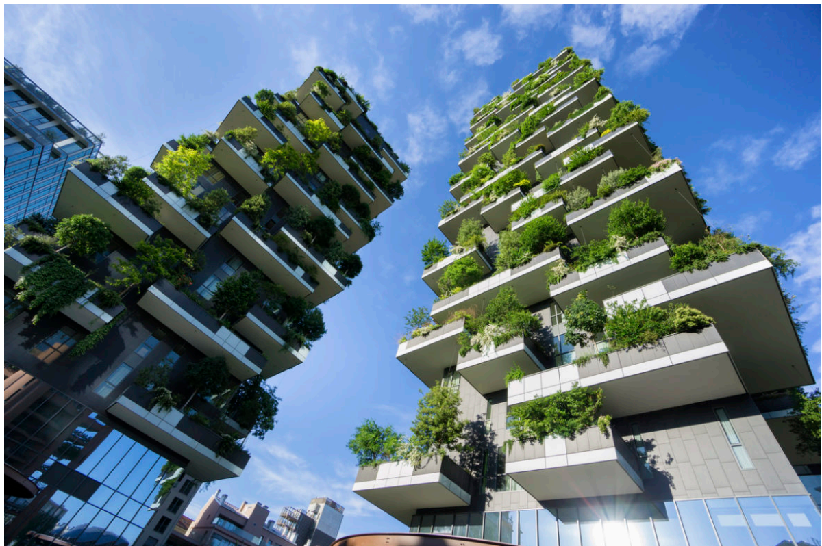
Figure 4.2: Bosco Verticale, residential building in Milan, Italy [79]
