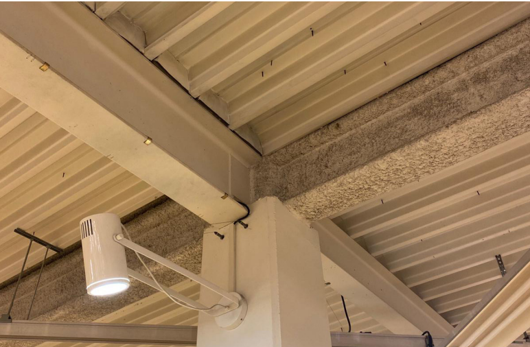
Steel beam on the concrete column
