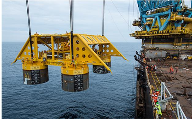
*Figure 2.1: Subsea template lowered through the wave zone, K. Aarset [2]*
