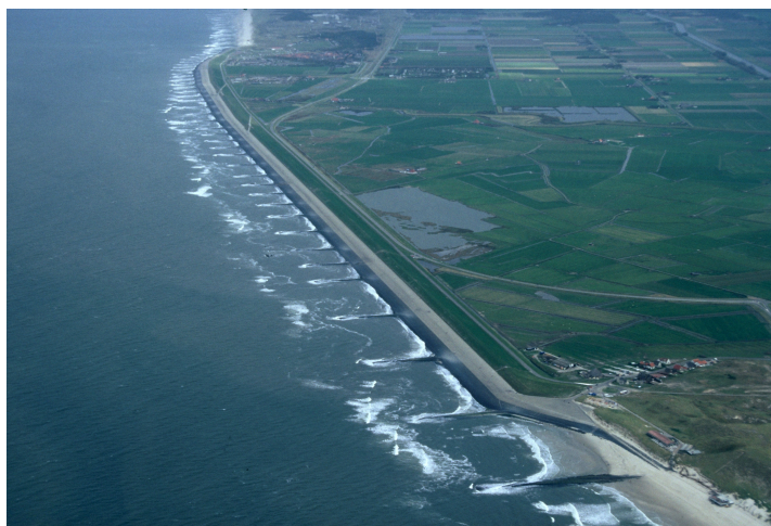
Figure 1.1: The Hondsbossche and Pettemer Sea defence before the implementation of the nourishment and thus the Hondsbossche Dunes (Rijkswaterstaat, 1985).
