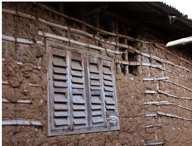
Appendix 7. Wattle-and-daub wall construction
