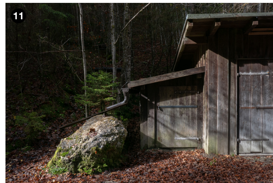
Rock gutter. A boulder becomes not only part of the façade of this storage hut, but supports the thin metal sheet guiding away the water from the building.
