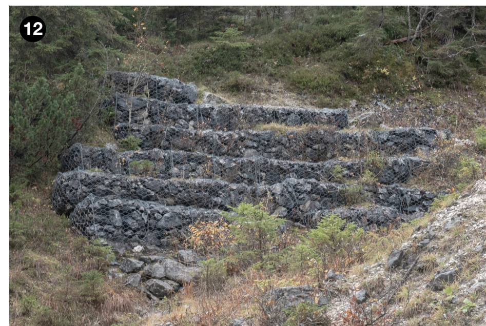
Path enforcement. Rocks sourced from the site are used to protect the steep slope below the path from erosion. Loose rocks are arranged into gabion walls, forming artificial horizontal layers within the naturally sloped landscape.
