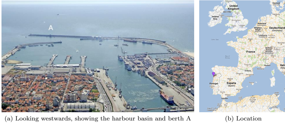
Figure 1.1: Location and overview of the Port of Leixões, Portugal
