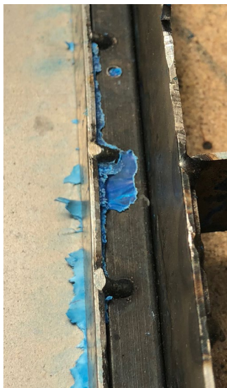
Figure 7-5, Plastic stuck on welds - Picture by Mark Bachrach
