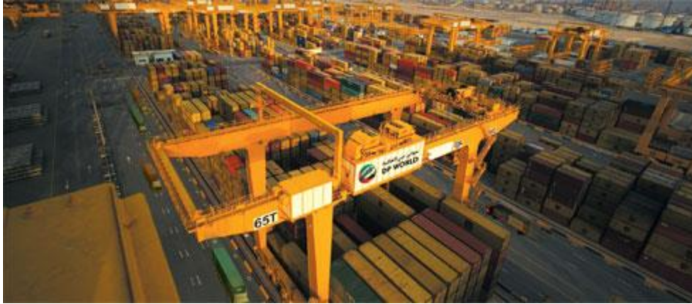
FIGURE L-4: RAIL MOUNTED GANTRY CRANES IN THE PORT OF JEBEL ALI, DUBAI (GULF PETROCHEMICALS & PETROCHEMICALS ASSOCIATION, SD)
