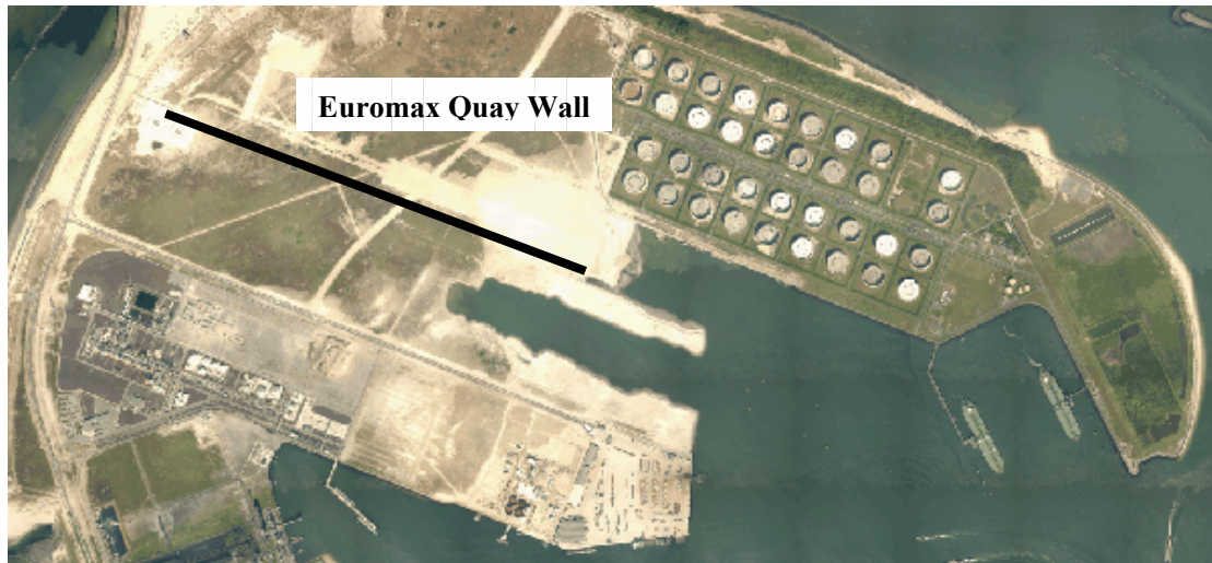
Figure 2-1: Yangtze Harbor in the Port of Rotterdam with top view on the construction area of the Euromax Quay Wall
