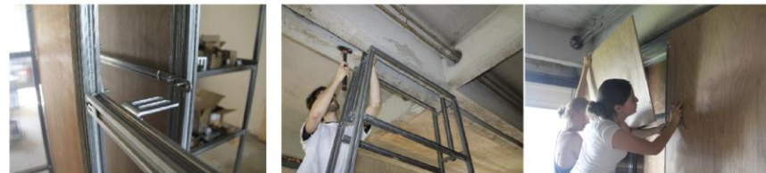
Figure 5. The steel frame wall with plywood panels.
