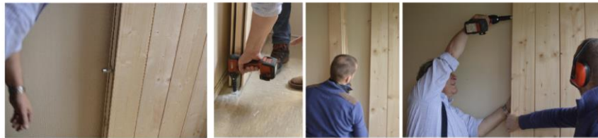
Figure 4. The massive wood interior partition wall.
