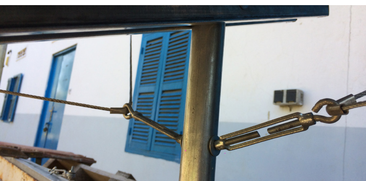
figure 92. Turnbuckle cable tensioner with (bent) butt connector
