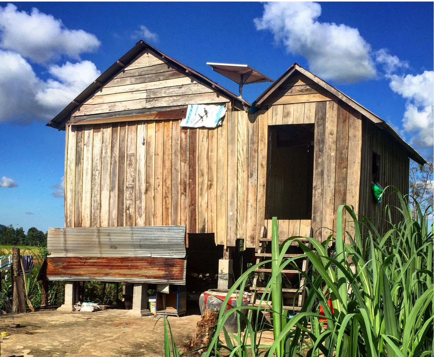
figure 59. An installed solar panel of the large SHS (© Kamworks)
