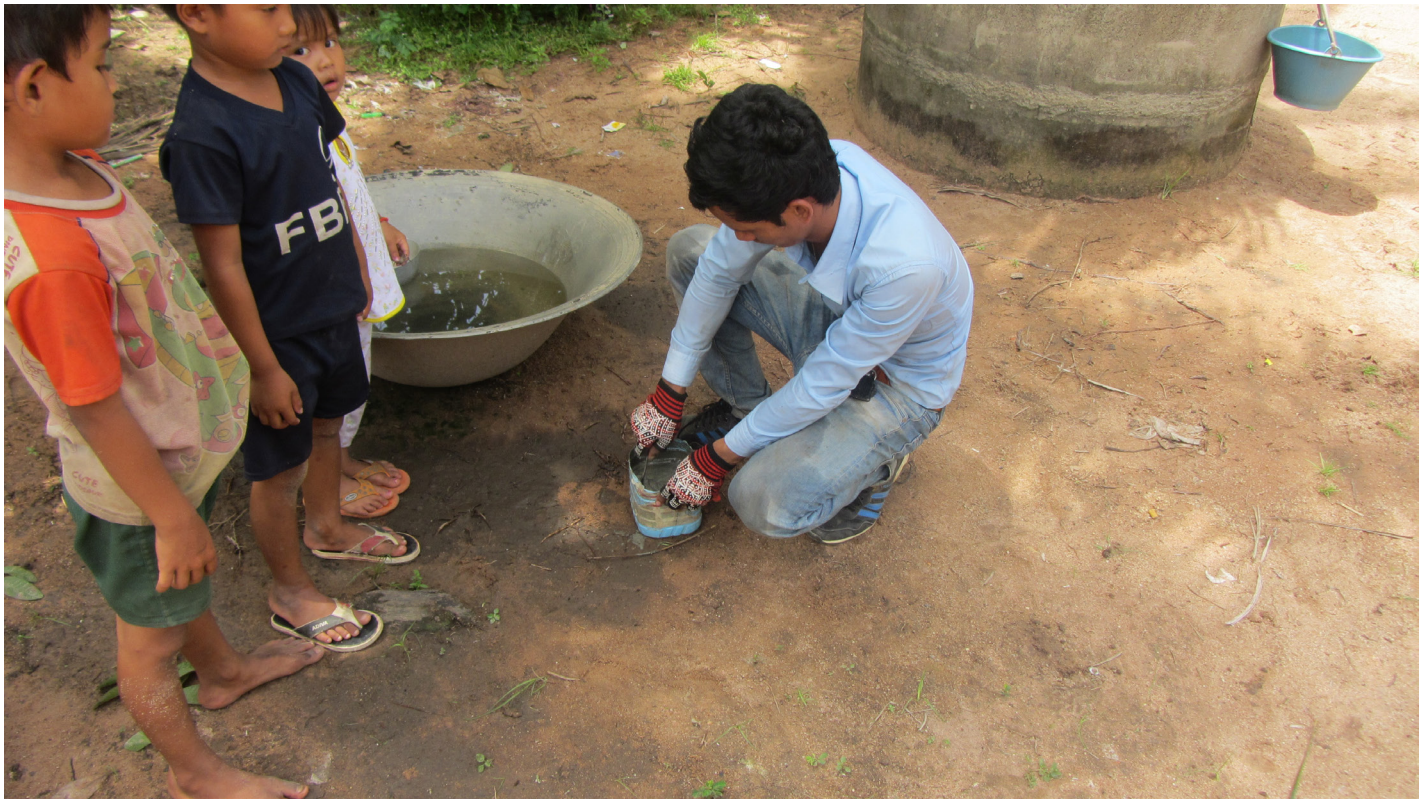
figure 66. A Kamworks technician making cement
