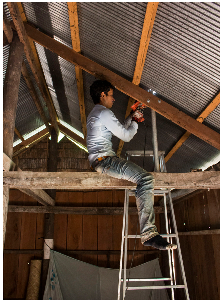
figure 75. Making a hole in the roof and mounting the pole
