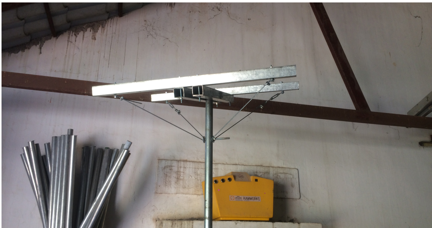
figure 88. The mounting pole with steel cables for increased stability
