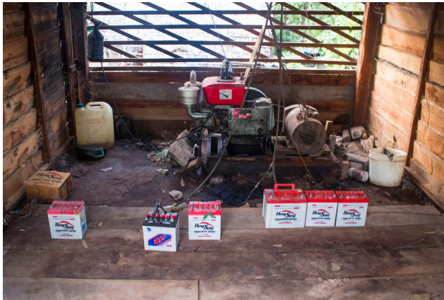
figure 12. Bringing a battery to the charging station
