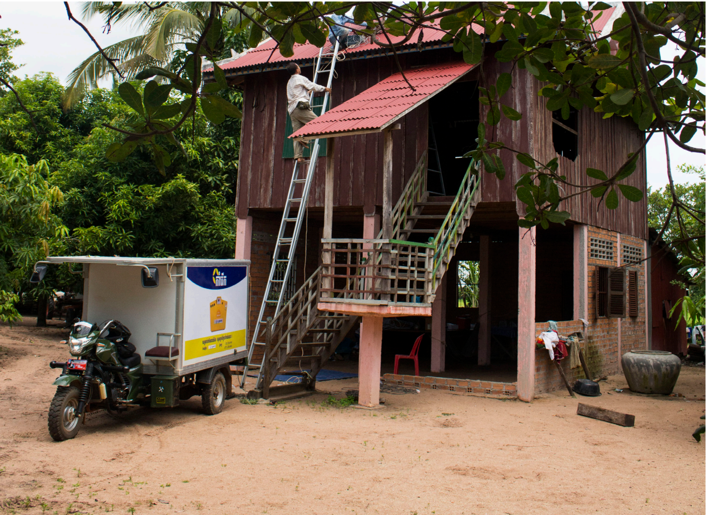
figure 7. One of Kamworks' TukTuks (left bottom) for transporting the Solar Home Systems
