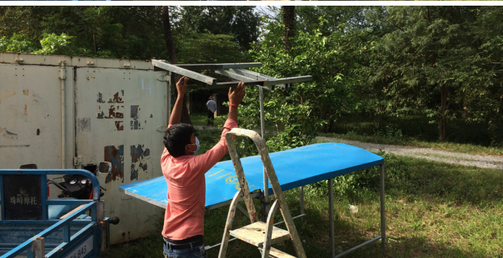
figure 86. Applying the expansion kit to the mounting pole
