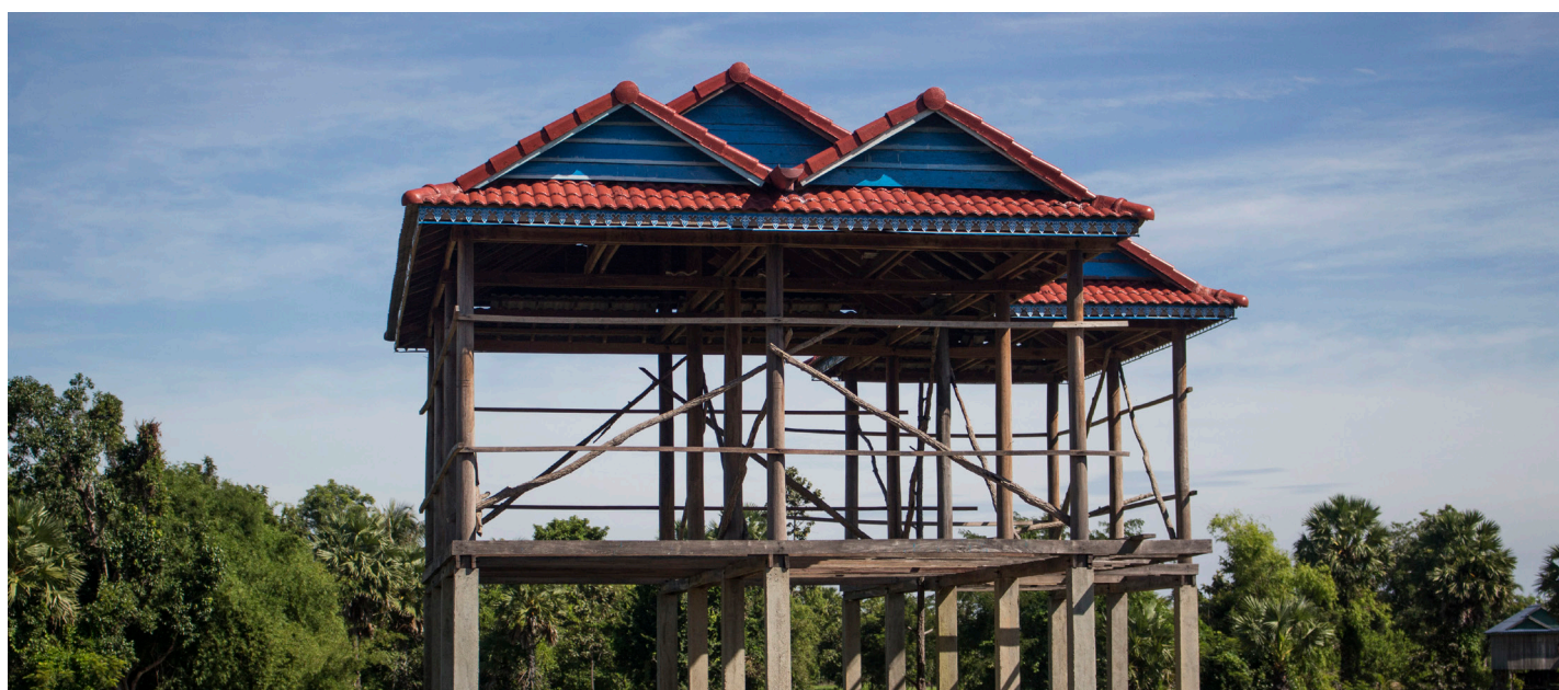
figure 64. Khmer house (in construction)
