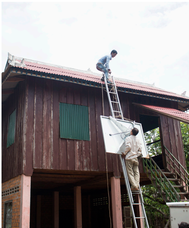
figure 73. Getting the panel with support on the roof
