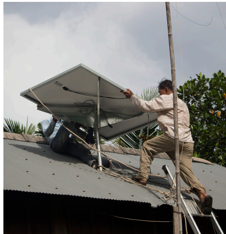
figure 74. Placing the panel support on the pole
