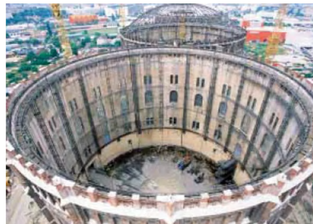
(2) Situation before reuse © Maria de la Paz.
