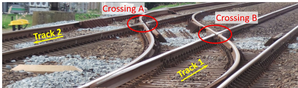
Figure 2.1. Typical crossover in the Dutch railway network.
