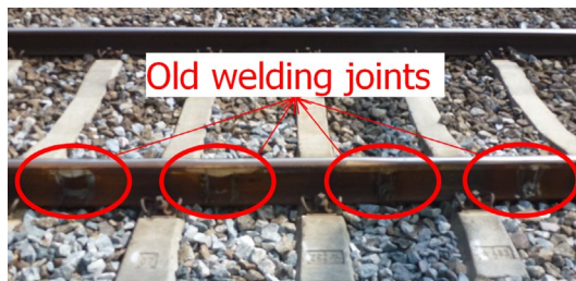
Figure 5.1. Welding joints test section.
