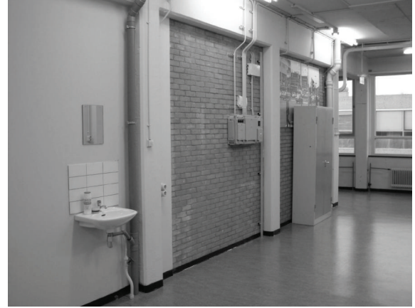
FIGURE 1: Photograph of the corridor wall.
