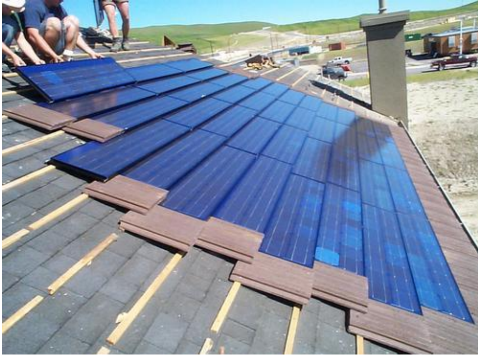
FIGURE 60: PV PANELS SHAPED LIKE A ROOF SHINGLE (CASEY & GRANT, 2013)
