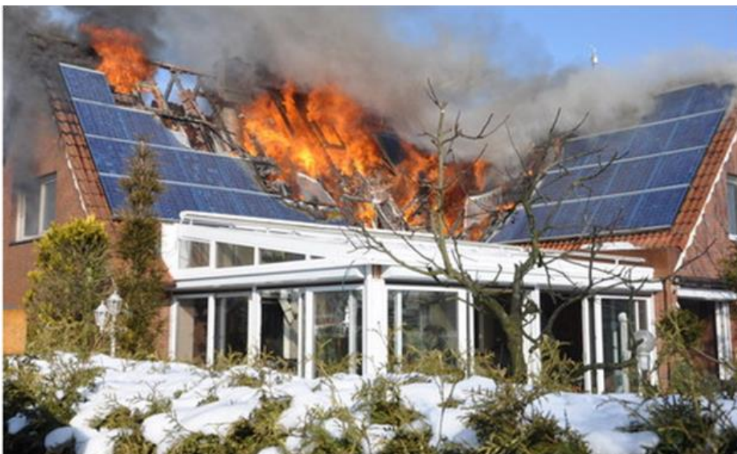
FIGURE 48: PV PANELS IN FIRE (BACKSTROM & DINI, 2011)
