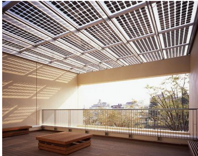
FIGURE 57: SEMITRANSSPARENT PV PANELS (SOLAR CONSTRUCTION, N.D.)
