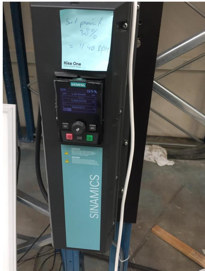
Figure A.6: Frequency converter to control pump RPM
