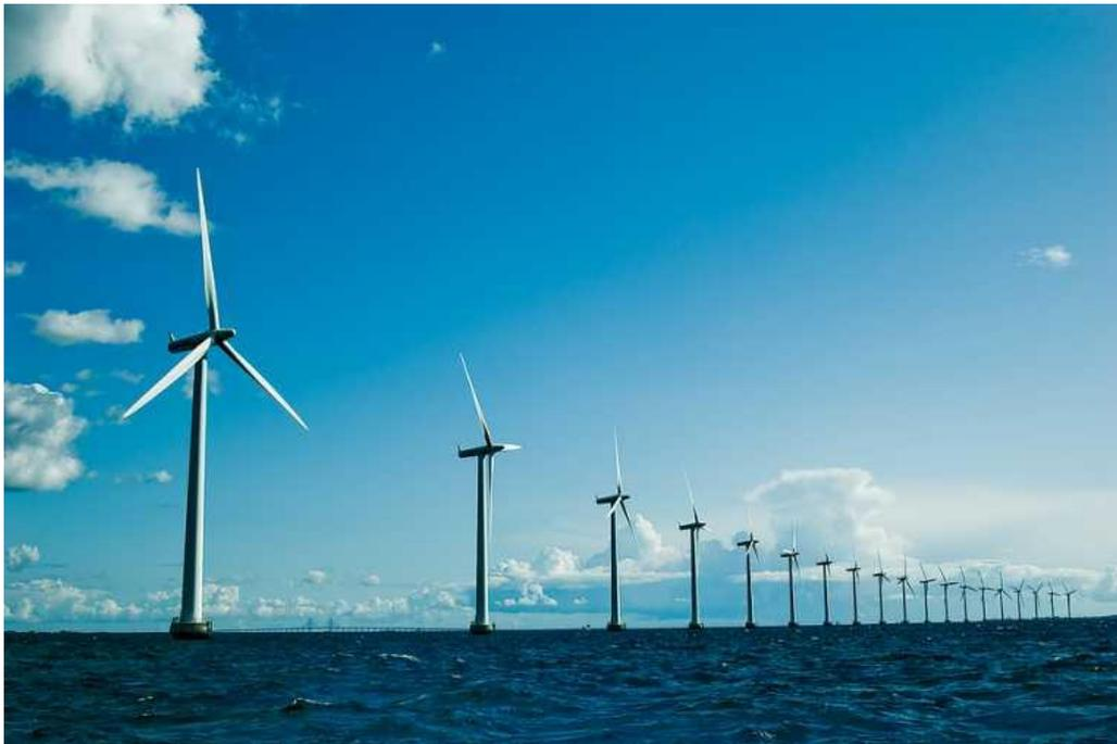
**Figure 3.1:** Part of Middelgrunden offshore wind farm, situated in Danish part of the North Sea. All turbines have a nominal power of 2MW and a total nameplate capacity of 40MW [1].
