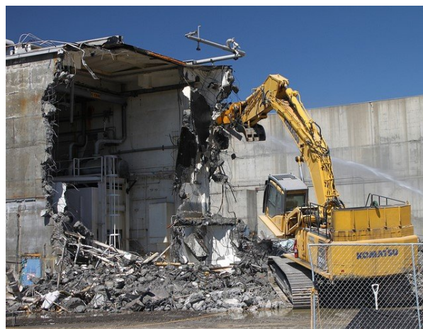
Figure 1.1: Demolition of a reinforced concrete building (EPA,2021, 2021)
