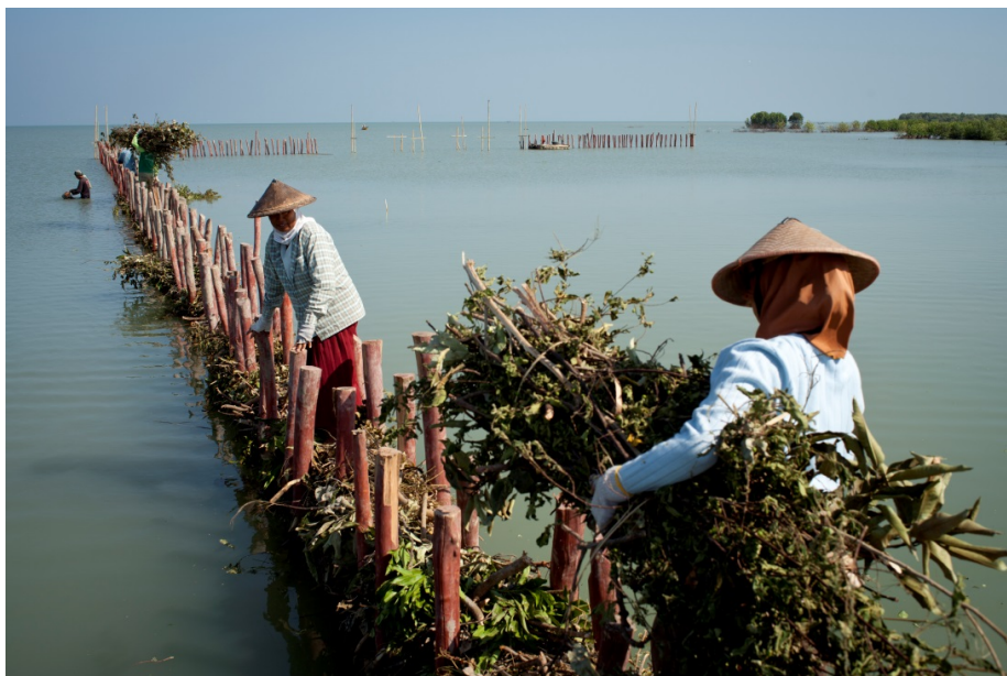
Figure B.7: Building of the permeable dams close to Demak, the pilot site for the Building with Nature solution [INFIS].
