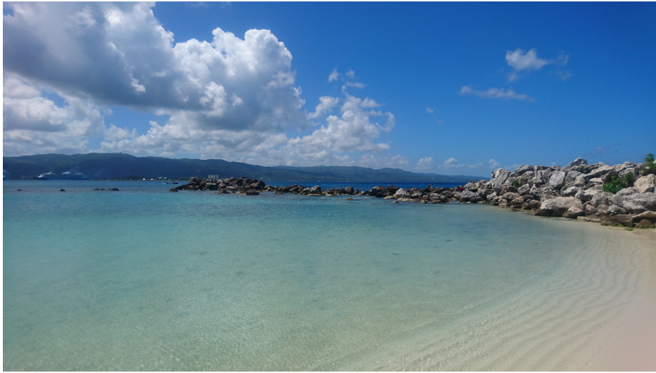
Figure A.3: Present state of the northern groyne.
