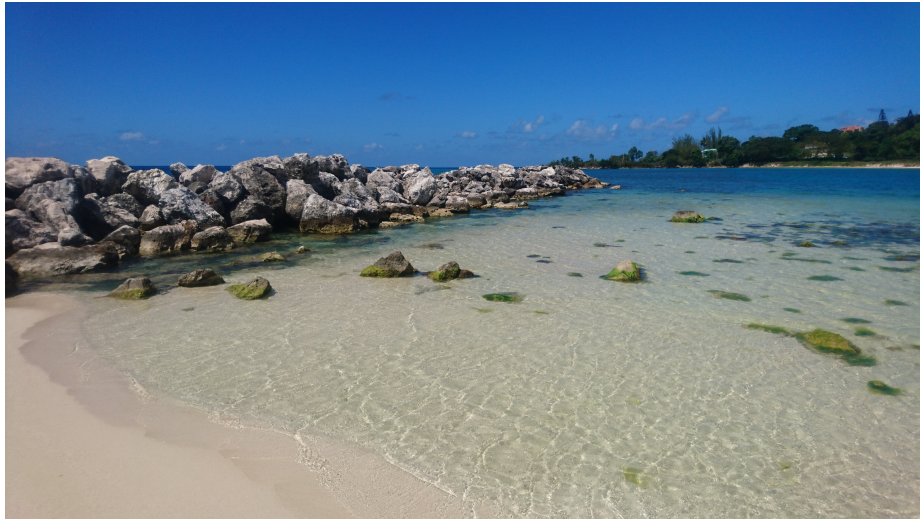
Figure A.13: Present state of the southern groyne.
