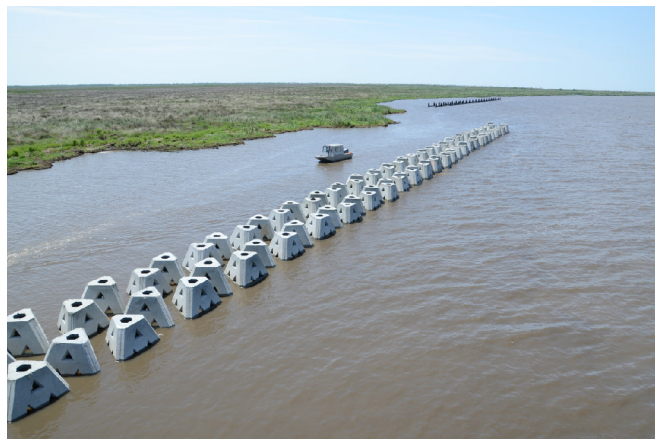
Figure 4.9: Wave Attenuation Devices (WADs) in sea. They emerge partly above water level.
