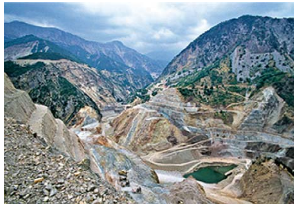
c: A view of Sykia dam.
