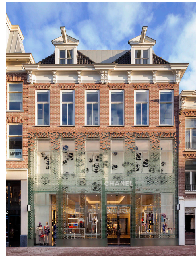
FIGURE 40: Figure showing Crystal House (Archdaily, 2016)
