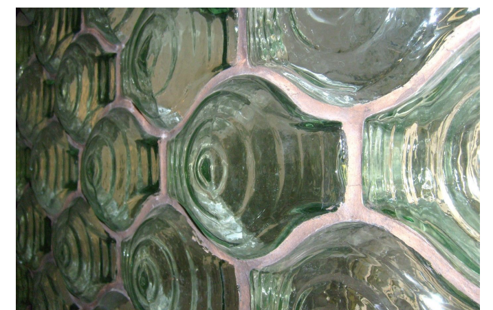
FIGURE 29 Figure showing installed Falconnier blocks (Glassian, n.d.)
