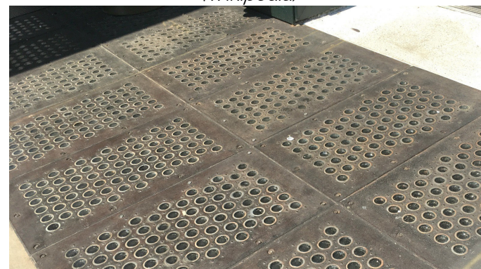
FIGURE 25: Figure showing Vault tiles (Paul. R, 2017)
