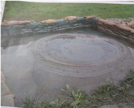
(a) Frequently reactivating sand boil near Guardia Ferrarese along the Po river, Italy [Martínez et al., 2020].
