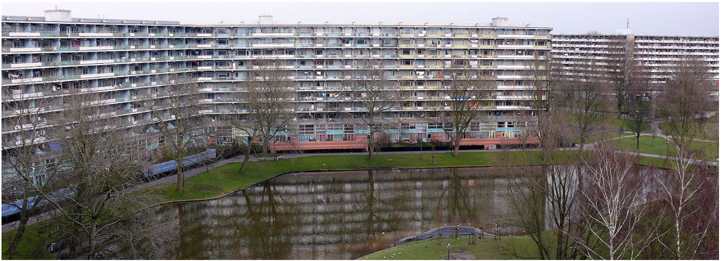
Fig. 4.40 - 'Gooioird' in the Bijlmer, Amsterdam. High-rises leave space for green but negatively affect microclimates, social control and parental attitudes, resulting in reduced outside play activity. Photo by Wikimedia user Hilton Teper.
