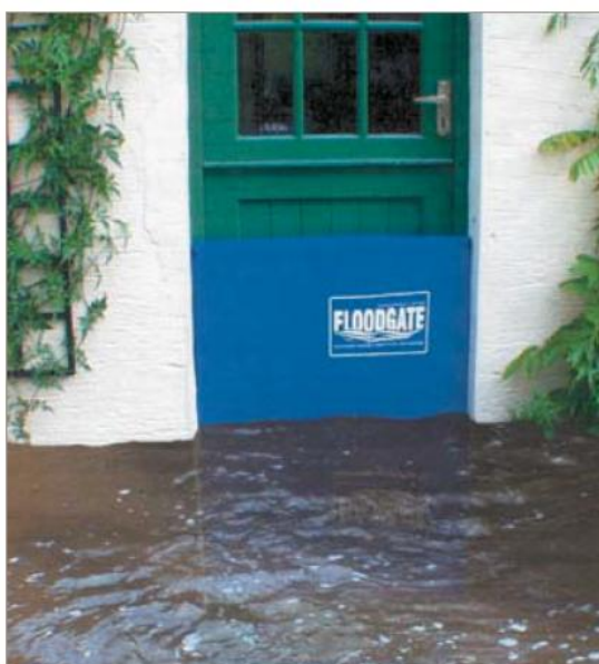
FIGURE 120: DOORWAY BARRIER IMPLEMENTED IN TYPICAL VIETNAMESE HOUSE (Bramley and Bowker 2002)
