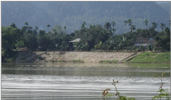
FIGURE 153: RIVERBANKS WITH NO PROTECTION STRUCTURES FOR FLOODING OR EROSION
