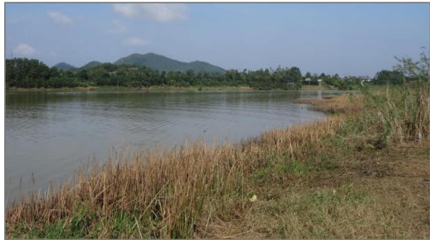
FIGURE 154: RIVERBANK WITH EROSION PROTECTION
