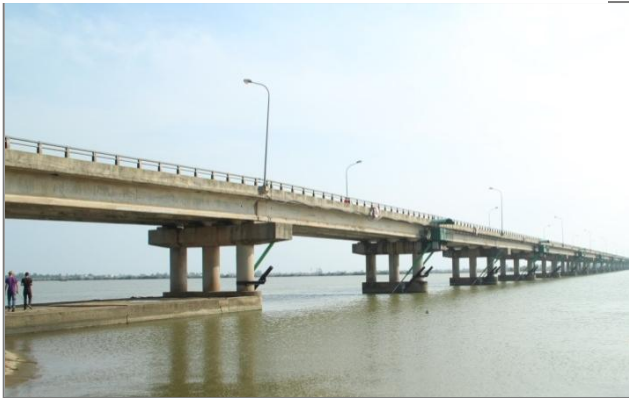
FIGURE 152: WEIR IN THE HUONG RIVER TO PREVENT SALT INTRUSION WHEN THE DISCHARGE IN THE RIVER IS LOW
