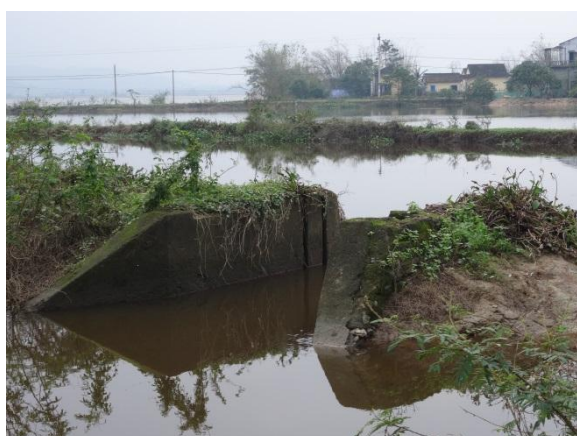
FIGURE 101: EXAMPLE OF A GATE IN A DIKE
