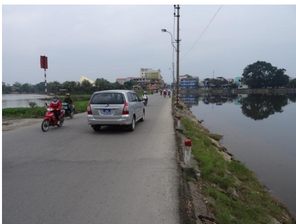
FIGURE 99: AN EXAMPLE OF A CLOSED OFF STREAM TO PREVENT SALT INTRUSION
