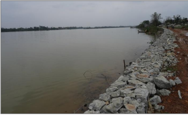
FIGURE 138: EROSION PROTECTION BY GABIONS ALONG THE HUONG RIVER
