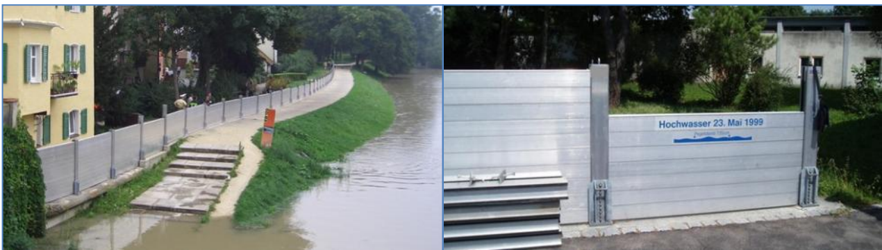
FIGURE 37: MOBILE PROTECTION SYSTEM IN USE IN GERMANY (RUNDFUNK 2013)
