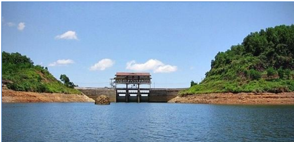
FIGURE 150: A SPILLWAY OF THE TRUOI RESERVOIR
