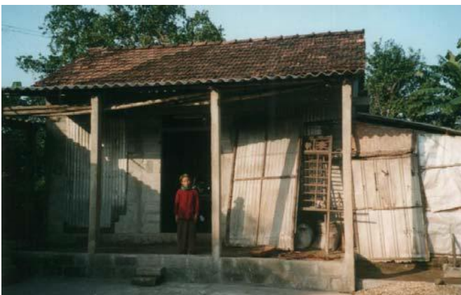
FIGURE 107: NON-TYPHOON PROOF HOUSE (NORTON AND CHANTRY 2002)
