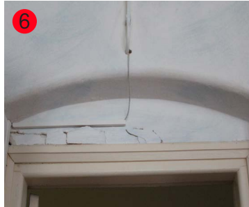
Image 176 Cracking in the arched part of the doors
