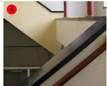
Image 136 Handrail, main staircase
