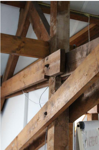
Image 60 Construction St. Jozef
