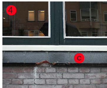
Image 112 Window lintel and sill
