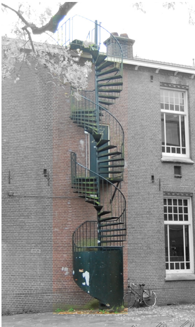
Image 11 Fire escape staircase on the north facade of the St. Anna (own photo, 2017)
