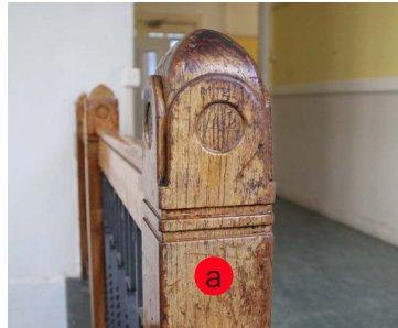
Image 146 Handrail, main staircase
