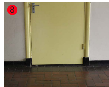
Image 140 Plinth, first floor
