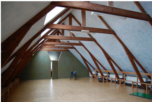
Image 62 Construction St. Anna (Own Photo)
