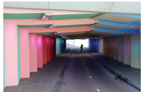
Image 52 Kostverlorentunnel (Own Photo)
