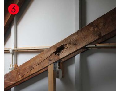
Image 162 Fracture on wooden beam
