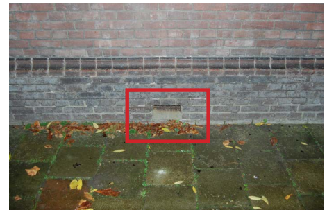
Image 181 Air inlet in facade (Own photo)
