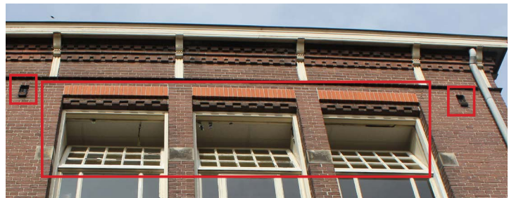
Image 184 Natural ventilation, air inlet in facade (Own Photo)
